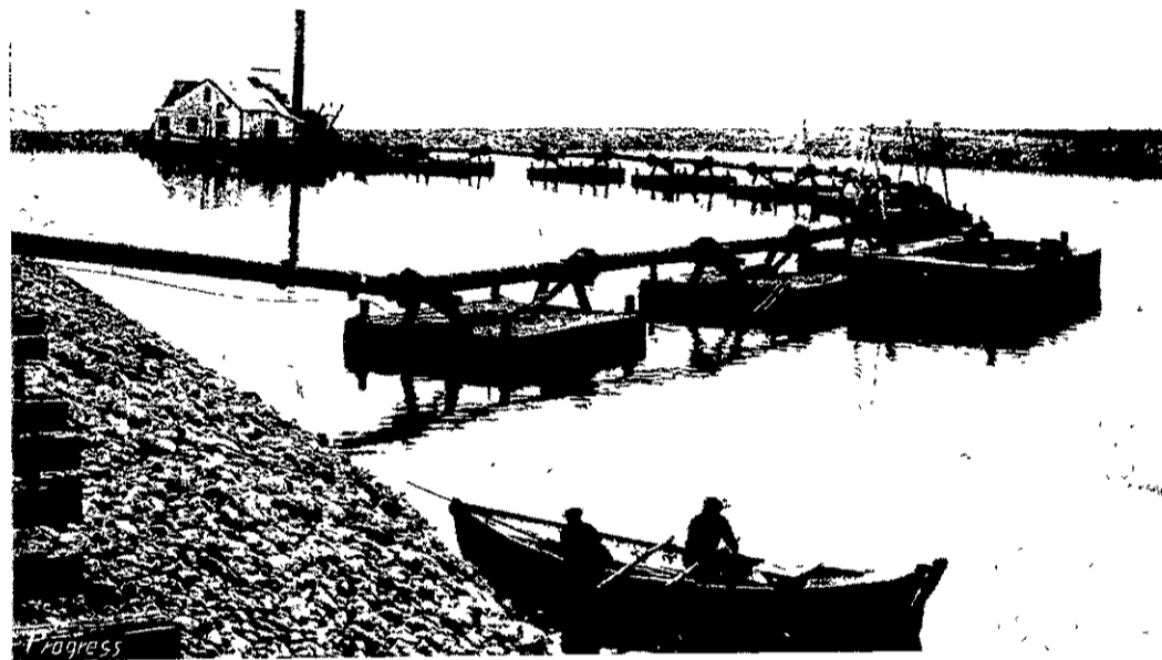
THE DREDGE AT WORK, NELSON HARBOUR IMPROVEMENTS.
