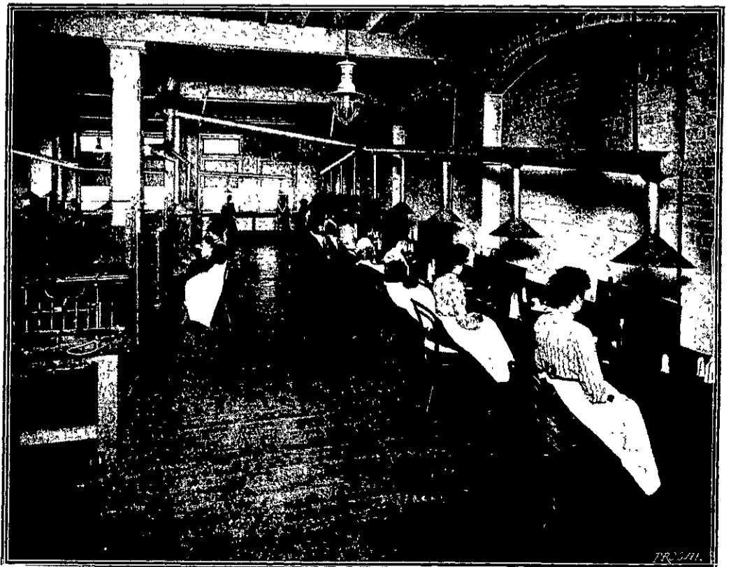
BURNING-OFF AND SHAPING THE MANTLES
