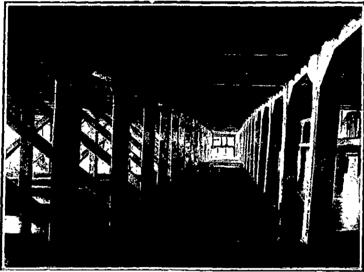
FERRO-CONCRETE WHARF CONSTRUCTION, AUCKLAND: UNDERNEATH VIEW.
