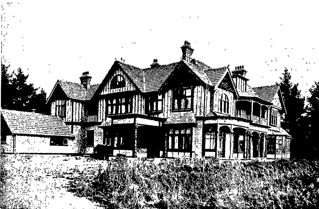
THE RESIDENCE OF MR. CRACROFT WILSON, CHRISTCHURCH.
