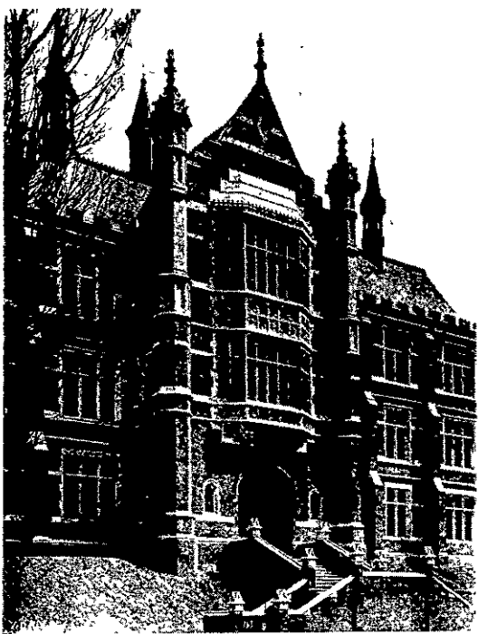
THE MAIN ENTRANCE. — THE ORIEL WINDOW OVER THE DOOR LIGHTS THE COLLEGE LIBRARY. THE TWO SIDE ROOMS BEING ALSO USED AS STACK ROOMS FOR BOOKS. THE ROOM OVER THE LIBRARY IS A MEETING-ROOM FOR THE STUDENTS' CLUBS.
