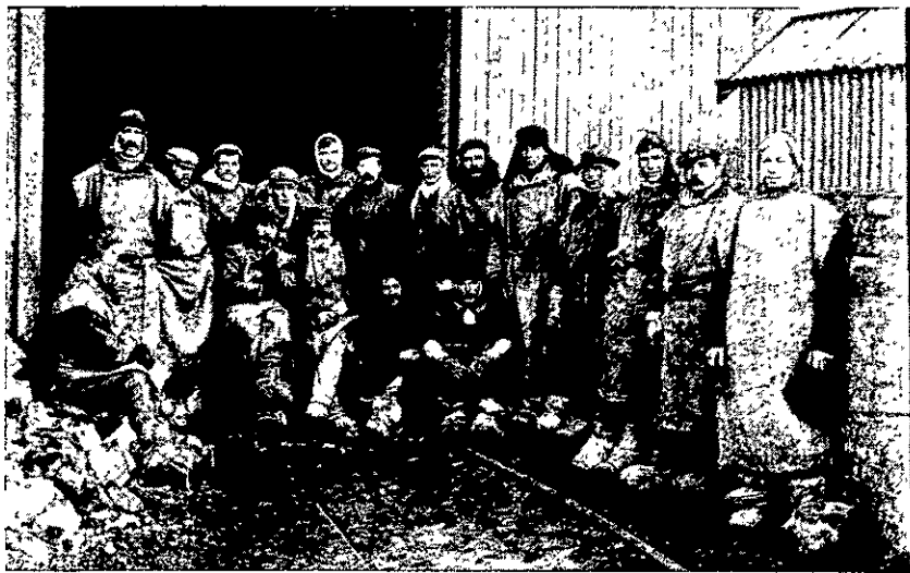
GEAR WORKS: EQUIPPED FOR WORKING IN THE FREEZING CHAMBER.
