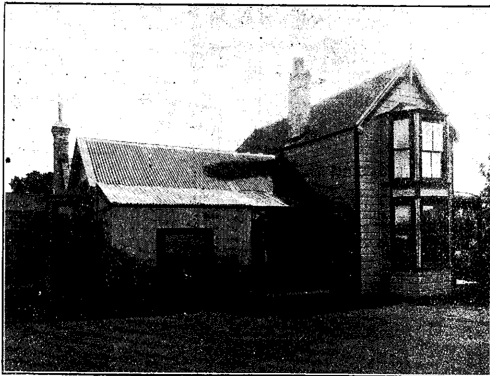
FIRST CATHOLIC CHURCH AND PRESBYTERY AT HAWERA. SHOWING ADDITION of TWO-STORIED BUILDING ERECTED by FATHER RYAN
