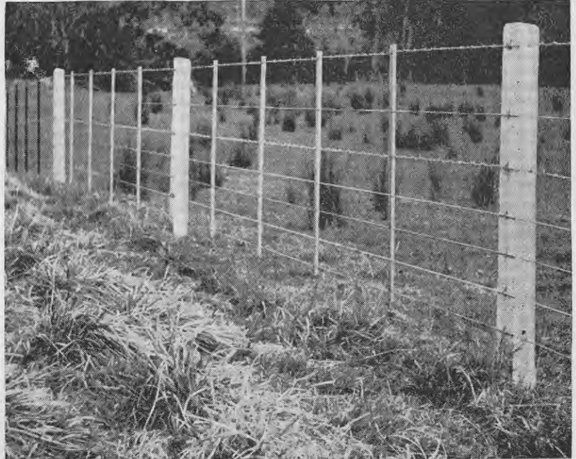
A typical concrete post and galvanised batten fence with No. 8 and barbed wires.
