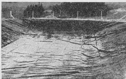
Garnite Moisture Barrier Film liner in position for 150,000 gallon reservoir.
