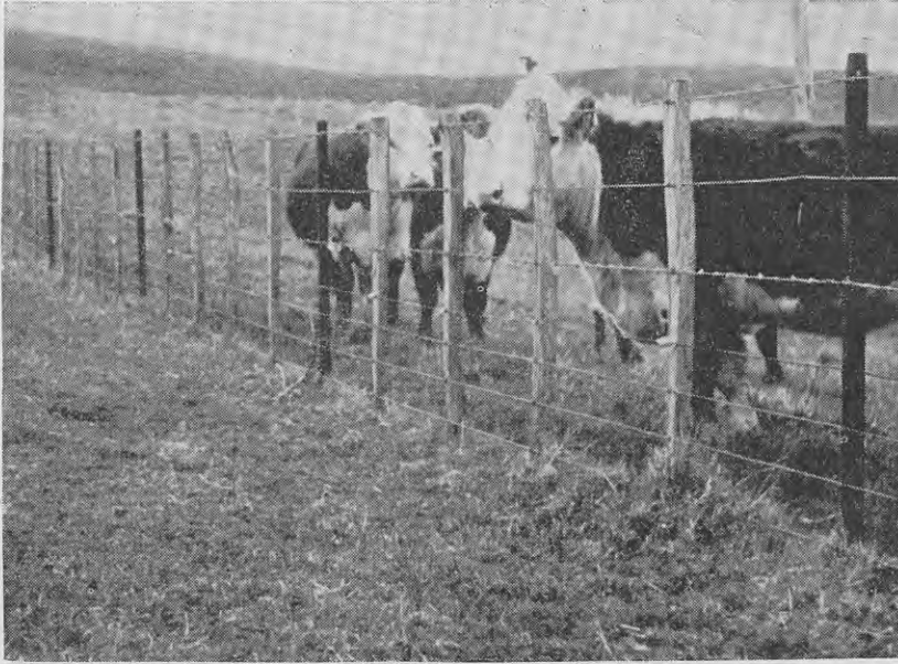
A seven-wire H-section steel post and wooden batten fence.
