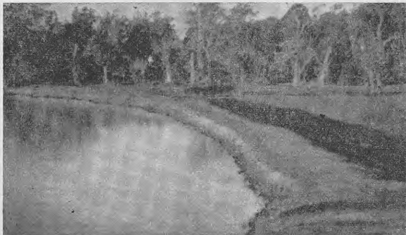
A "turkey nest tank" nearly filled at the McGarvie Smith Animal Husbandry Farm of the University of Sydney. The creek from which the water was pumped to fill the dam runs among the trees in the background.
