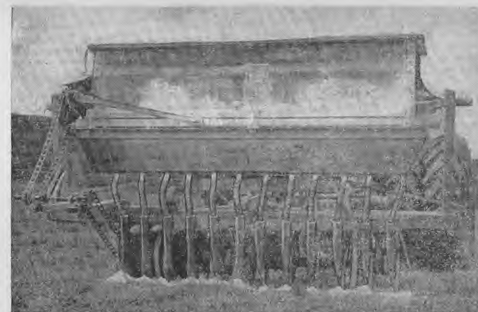
The "White" disc-seeder. Seed and fertiliser are mixed together and then sown through the distributor mounted above the discs. Tubes guide the mixture into the grooves left by the slightly angled discs. The wheels placed between the second and third blades at each end prevent excessive penetration, even though the disc blades may be angled sufficiently to scoop out an almost clean groove.
