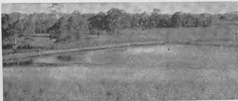
Part of the animal husbandry farm, showing a dam which was recently constructed for harvesting water for irrigation. The only earthwork required was the bank in front of the trees.
