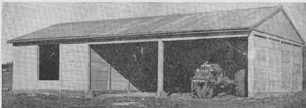
Buildings should be constructed with materials which will give greatest permanence with least maintenance. This implement and storage shed was built of foamed concrete units by 4 men in 8 days on a site 230 miles from the factory supplying the units. The cost was 10s. per square foot.
