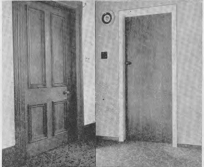
A contrast in finishing methods. Left—Panelled door, heavily moulded architrave, and high and heavily moulded skirting which were widely used 40 years ago. Right—Modern flush door with plain architraves and skirting.
