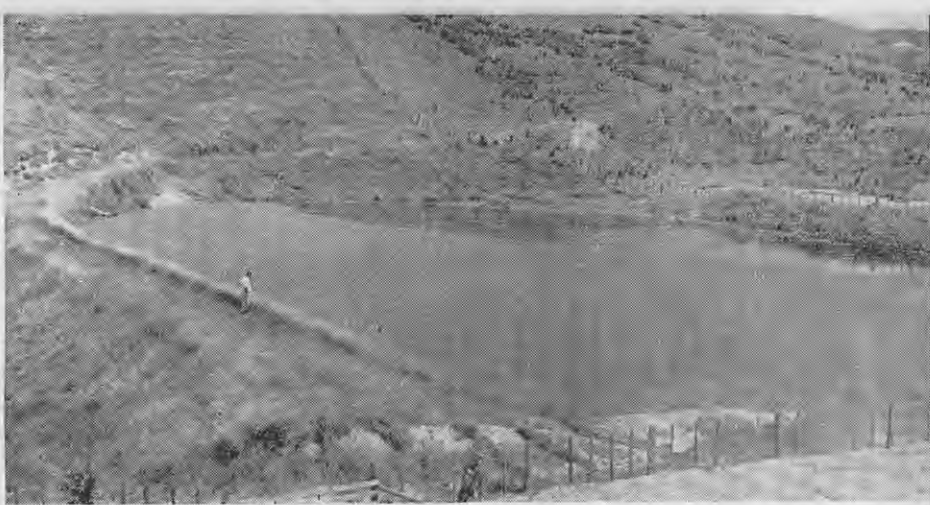
A dual-purpose water control dam in Poverty Bay. Such dams can be used for storing extra stock water and to supplement irrigation and fire-fighting supplies.
