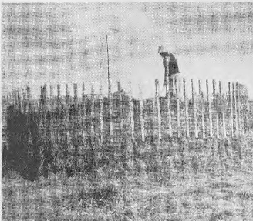
The fence has been raised for the first time and filling continues.
