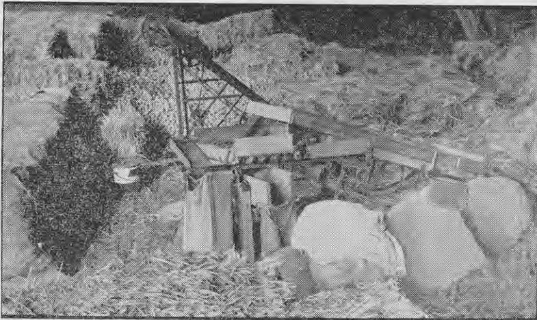
A grading and bagging machine ready for work at the pit.
