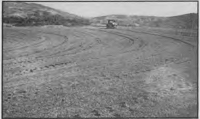
Guide lining rolling clay downs.
