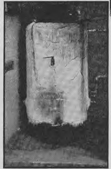
Steam boilers should be installed in separate fire-proof rooms of honey houses.
