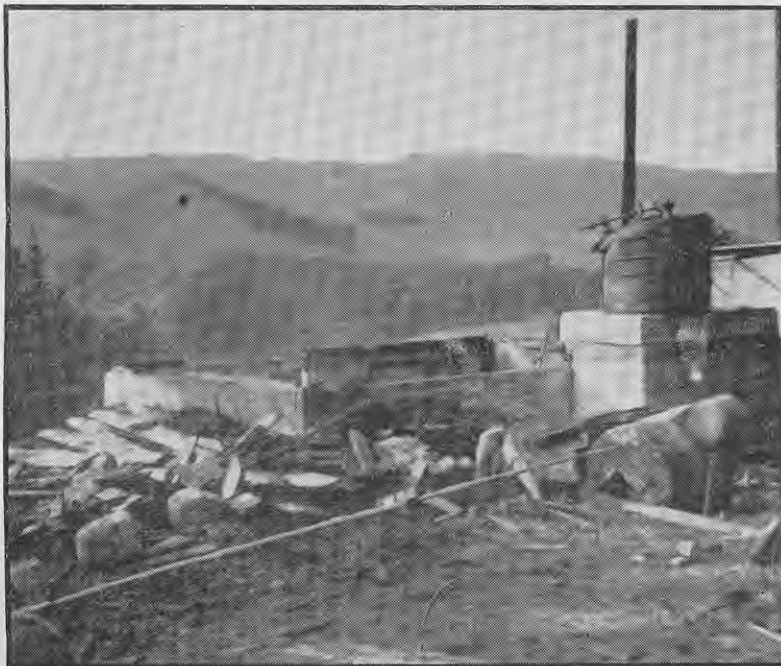
It is suspected that a defect in electrical equipment caused the fire which destroyed this honey house.
