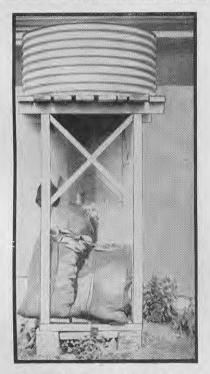
It is possible even with a rain-water tank, if it can be placed high enough, to obtain adequate pressure for a piped interior water supply. However, this small storage tank would not supply the house for more than a few days without rain.
