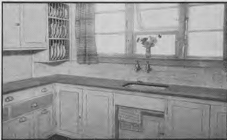
Unlimited hot and cold water, under pressure and at the turn of a tap, is one of the greatest labour savers that modern engineering and plumbing can make available to even the most remote farm home.
