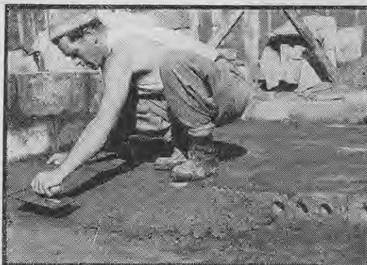
Above—The Division's engineering section advises on farm structures, farm mechanisation and mechanics, and water supplies. Right—The forestry section fosters the judicious planting of hedges and shelter and timber trees.
