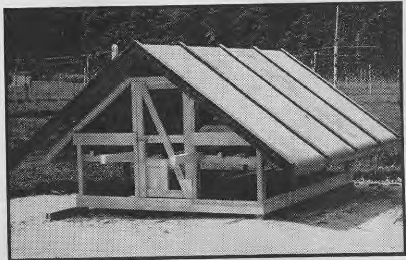
A colony house which is suitable for the housing of growing pullets. This type of house is portable, adaptable to weather conditions, and cheap and simple to construct.
