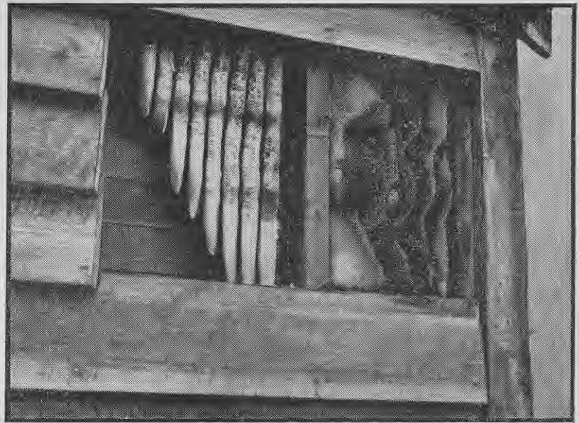
New comb (left) and old comb (right) in a farm building. The clean, diagonal cut through the weatherboards will simplify replacement of them neatly. Wild bee comb in a wooden building is usually found attached to the top plate and built down between studs.
