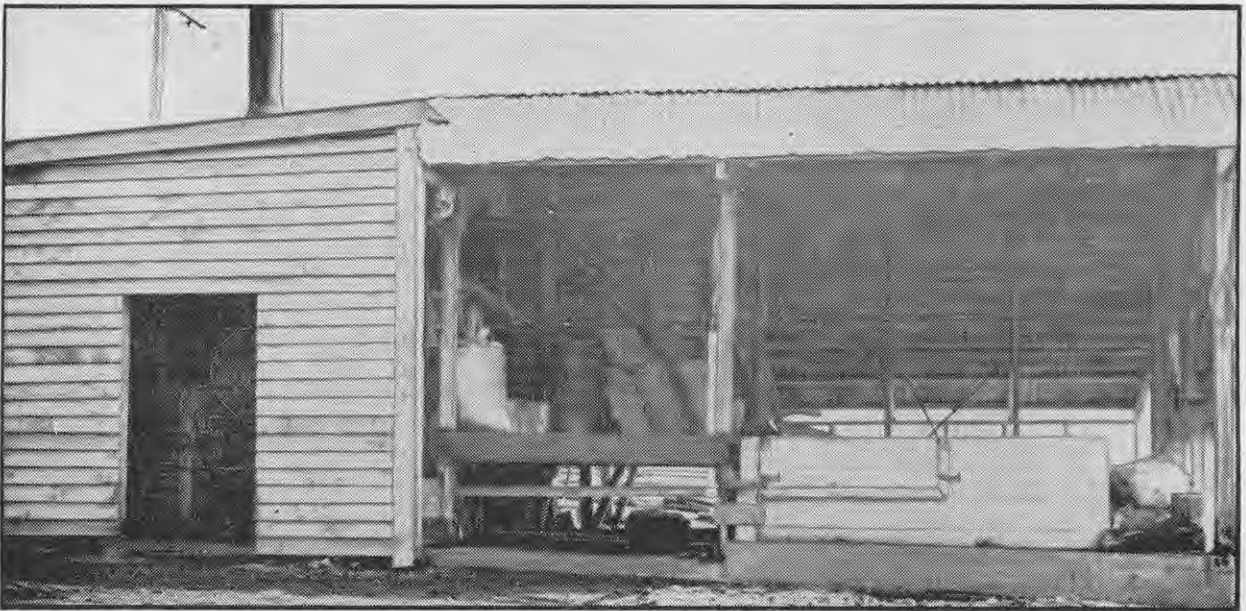
Front of boiler house, showing landing stage (middle) and concrete sterilising vats (right).
