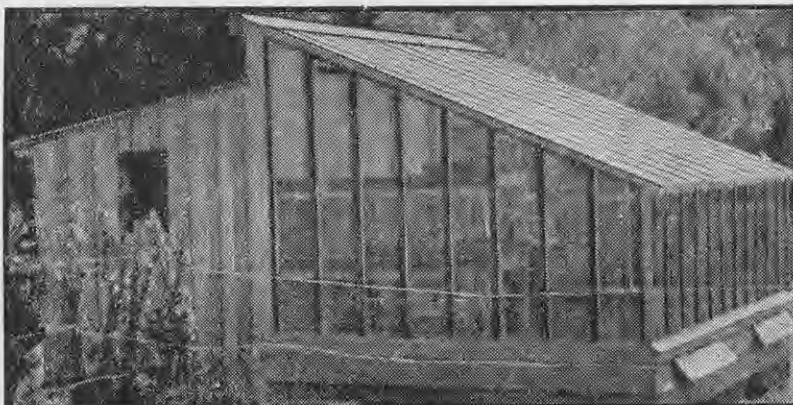
A type of frame not often seen. Built like a miniature glasshouse, it has some advantages of a glasshouse together with those of a frame. It can be heated readily with a kerosene- or oil-burning heater.
