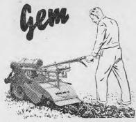
Differential lock reduces fatigue— There's no wrestling with a Rotavator "Gem". Differential ensures easier turning on corners and tricky headlands.
