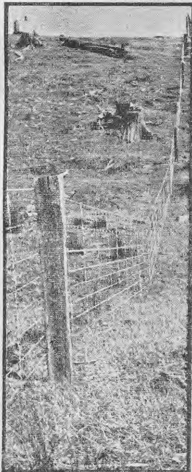
Fig. 2—Hunter fence, showing in foreground span of 30yds. without posts.
