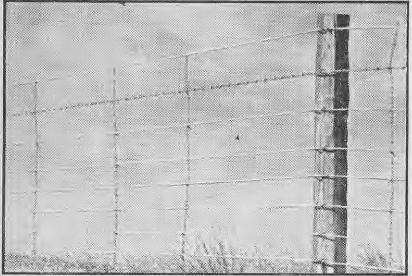
Fig. 1—Hunter fence showing battens replaced by chain. Plain wire is shown on the bottom, but this has since been replaced by barbed wire.
