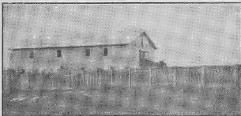
Fig. 6—An all-concrete fence is permanent and upkeep is low.
