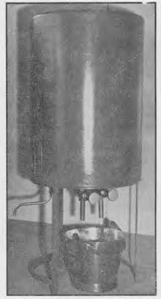
Modern type of dairy water heater in which the cylinder is lagged with \$\frac{1}{4}\$in. asbestos sheeting. Two draw-off pipes and the overflow discharge are under the cylinder. Power is cut off by thermostat control only when the water boils, and loss of heat between milkings is negligible.
