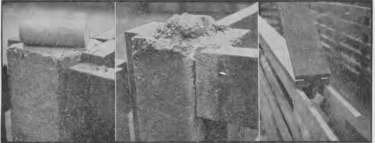
Fig. 14—Riddle exposed to the weather soon disintegrates. A simple remedy is to build a cupboard (right) into the double dividing fence of the crush pens.
