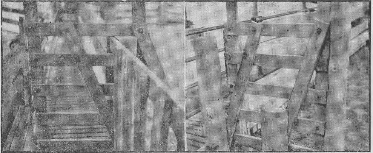
Fig. 11—"Disappearing" gate, shut (left) and open (right).
