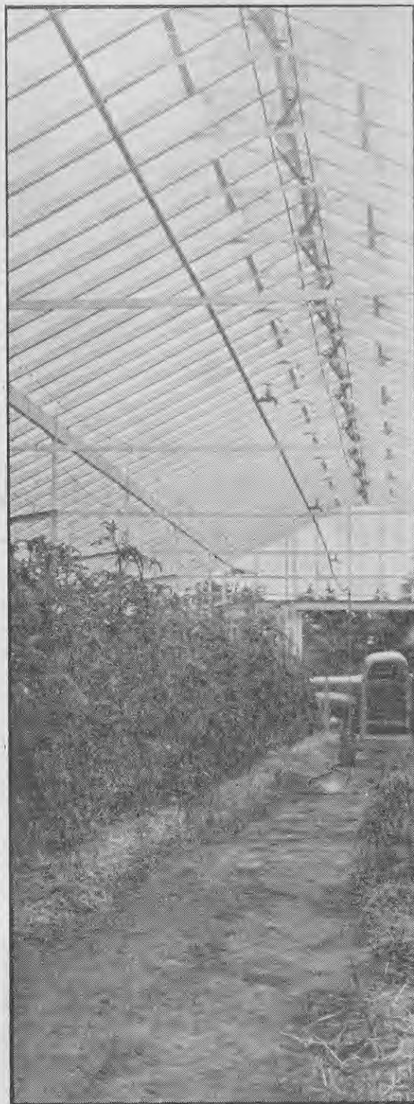
The ventilators fully opened.
