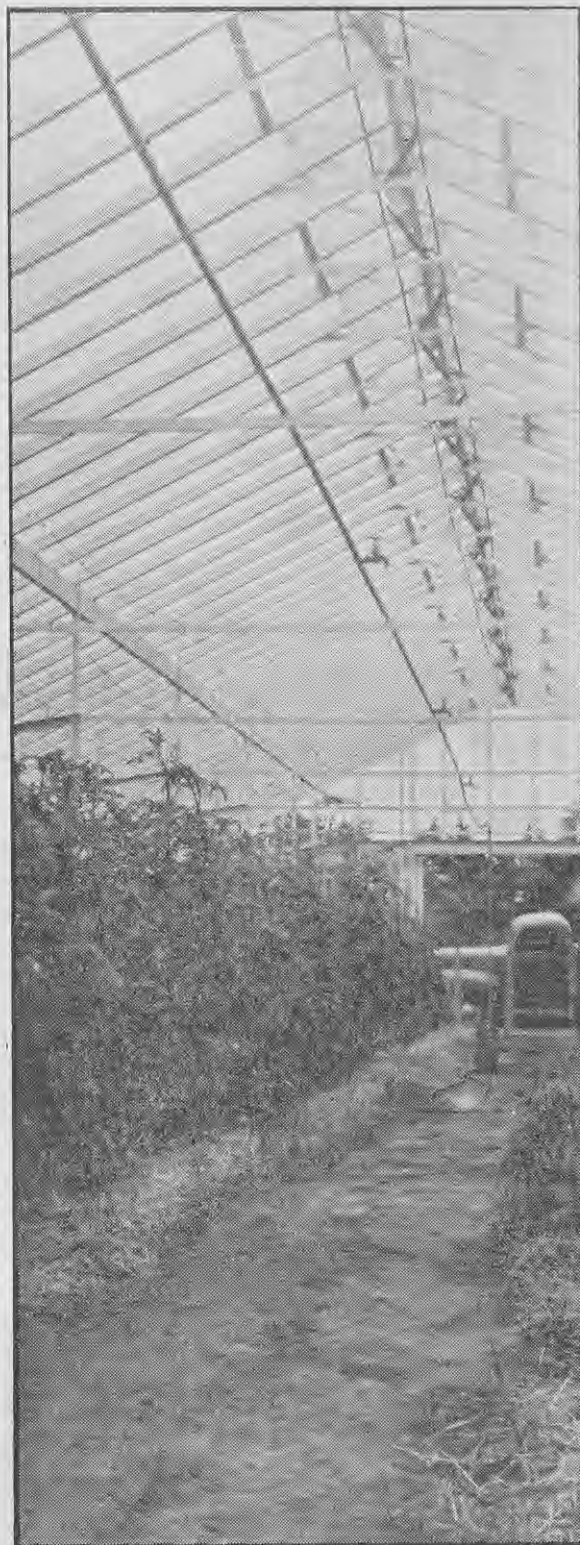
The ventilators fully opened.
