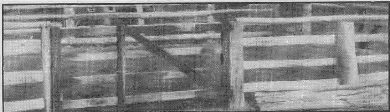
A stockyard built with posts of home-grown Robinia pseudacacia and rails of Eucalyptus obliqua .
