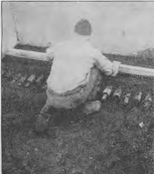
After more mix has been put on it is screeded to give a 1in. cover over the mandrels.
