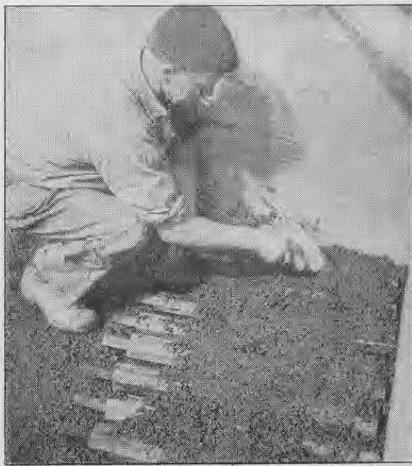
Left—Covering the mandrels with the mix. Right—Working the mix in between the mandrels. The space between the ends of the mandrels and the back wall is filled with concrete to block the ends of the cavities.
