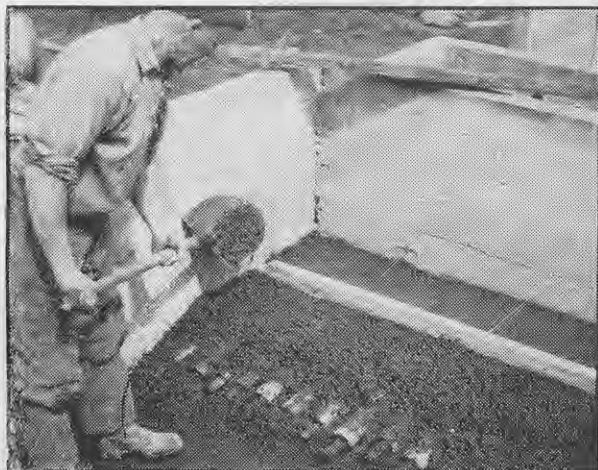
After having the mix worked between them the mandrels are covered again to complete the second section.
