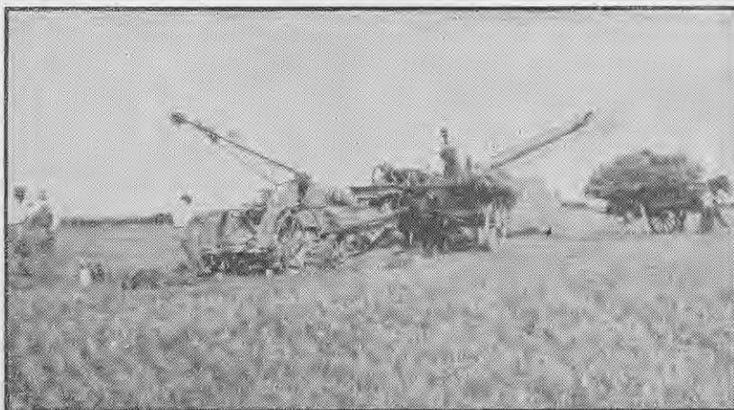
A threshing mill operated by an electrically-driven tractor.
