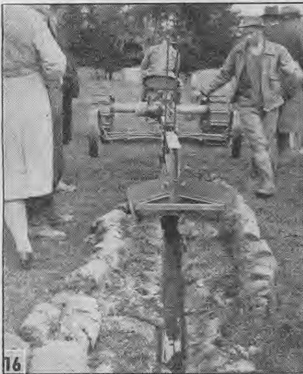
16. The Linton drain digger making the first cut, of 5 to 6in., by a special blade which is regulated for depth at each cut. 17. The Linton machine entering the end of the drain for the second cut, which is made by a sharp scoop and slot through which the soil is forced into an inclined slide which fits the trench. Seven to eight cuts are required for the full depth of 36in.
