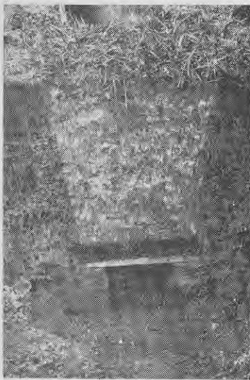
A slab drain made by cutting a narrow channel in the bottom of a drain and placing a wooden slab across the shoulders.
