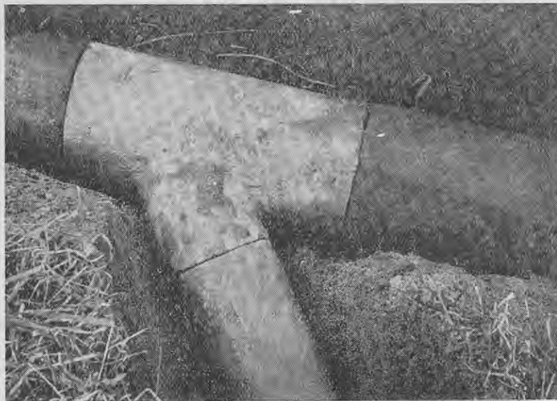
Subsidiary drains should enter main drains at an acute angle and properly-made junction tiles should be used.
