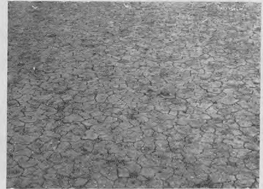
Cracking which takes place on sandy loam areas after tide water has been shut off by stopbanking. These areas are easy to drain and are in a condition for grassing 2 to 3 years after stopbanking.
