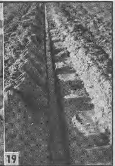
18. The Linton machine in action. The spoil is lifted up on the slide bar and is pushed to either side by the wings fitted to the rear of the frame. 19. A completed drain ready for grading and bottoming as dug by the Linton ditcher on a Manawatu farm. The shaped cutter and scoop reduce to a minimum the work required to finish the drain.
