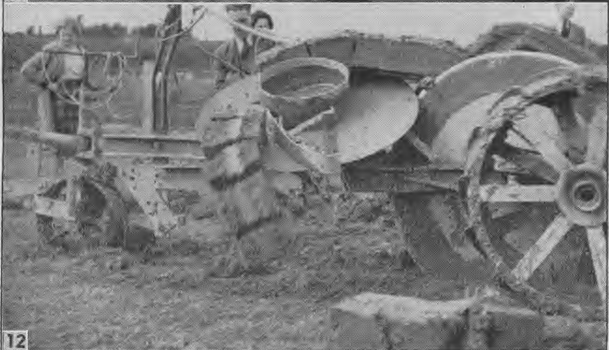
11. The revolving disc which carries the spoil 5 or 6ft. clear of the side of the drain, leaving plenty of room for the machine to operate in successive runs along the drain. 12. The discharge of spoil from the Lewis drain digger. Note: Both the cutting discs and the conveyor disc work by friction only. There are no gear-driven parts on the machine.
