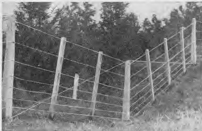
Fig. 15—Method of fastening down a post in low place where the land is wet. Two strands of No. 8 wire are fastened at ground level to each side post planted on solid land, and passed over the top of the post in the hollow, and tightened by twisting with the two pieces of wood.
