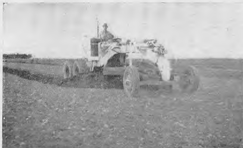
Construction of border for border dike system.
