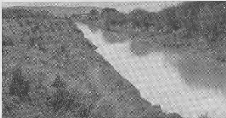
On low-lying country drainage plays an important part in the elimination and control of weeds, such as nigger-head and rushes. Here is shown the outlet drain of a large drainage scheme in Otago.
