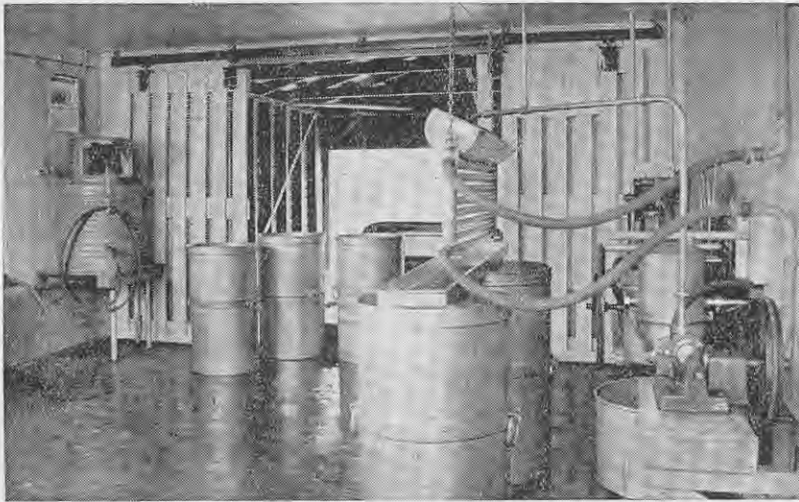
Fig. 3.—Milk-room of shed shown on page 217. Floor built up to floor level of delivery truck, and roof extended to provide cover for truck. Note vertical lining.
