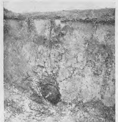
Fig. 4.—When the back plate strikes the bank the pipe is automatically released from the mole plug.
