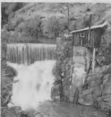
Fig. 15.—A turbine-type generator. Note the draught tube down to the base of the dam, allowing the plant to use a full head of water.
