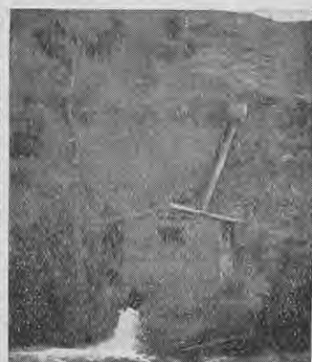
Fig. 16.—A large private power scheme in the Murchison district generating 12-15 h.p. (fall 31 ft.; flow 30 cubic feet per minute in pipeline).
