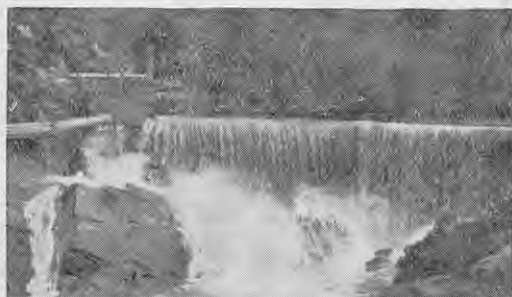
Fig. 14.—The concreted dam and intake (left) feeding the corrugated iron raceway to the water wheel.
