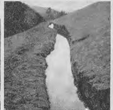
Fig. 8.—The intake raceway channelled along a hillside.
