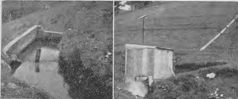
Fig. 9—The terminal point of the raceway concreted and with a wire screen from which water is led down by pipeline to the power house below. Fig. 10—The power house and water discharging to the valley floor.
