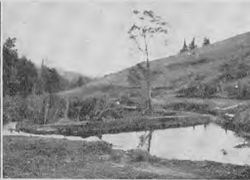
Fig. 7.—The reverse view, looking downstream, shows the dam with the raceway to the right and the spillway to the left.
