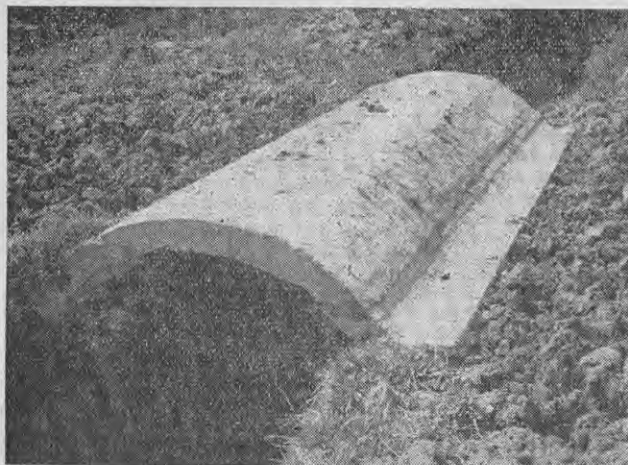
Fig. 7.—This illustration shows a bridge with the outer ledge resting on the hard sub-soil.
