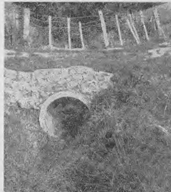
Figs. 4 and 5.—Alternative "facings" for retaining the earth covering. Fig. 5 provides a guarantee of strength.
