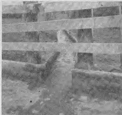
Fig. 2.—The type of drain recommended. This takes the washings well away from the shed.
