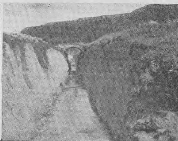
Fig. 8.—A bridge in miniature. This picture gives some idea of the size of the drain on Mr. McLean's farm.
