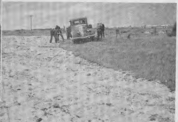
Stripping turf from shell beds.
