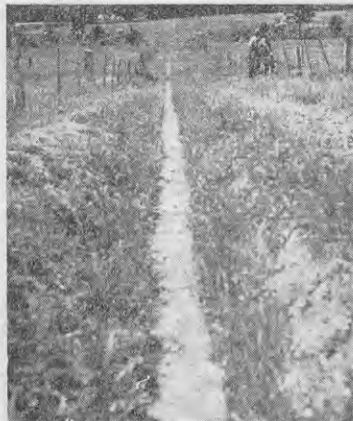
Pugging of the cow race may be overcome by constructing a concrete walk. Although only 18in. wide, this walk has proved highly effective.
