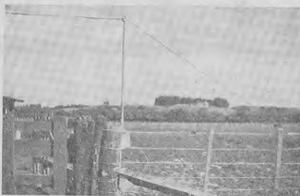
Left: The electric gateway. Right: Carrying the electric wire overhead. Note the length of old piping. The insulator is attached with a doubled loop of No. 8 fencing wire split pin-fashion.
