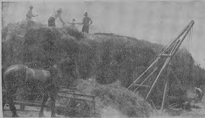
The fork type of elevator with the wheeled sweep in action.
