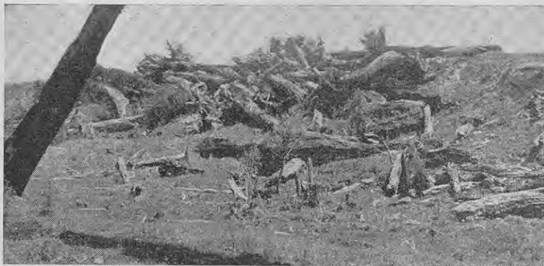
Logs dragged over the bank with a tractor.
