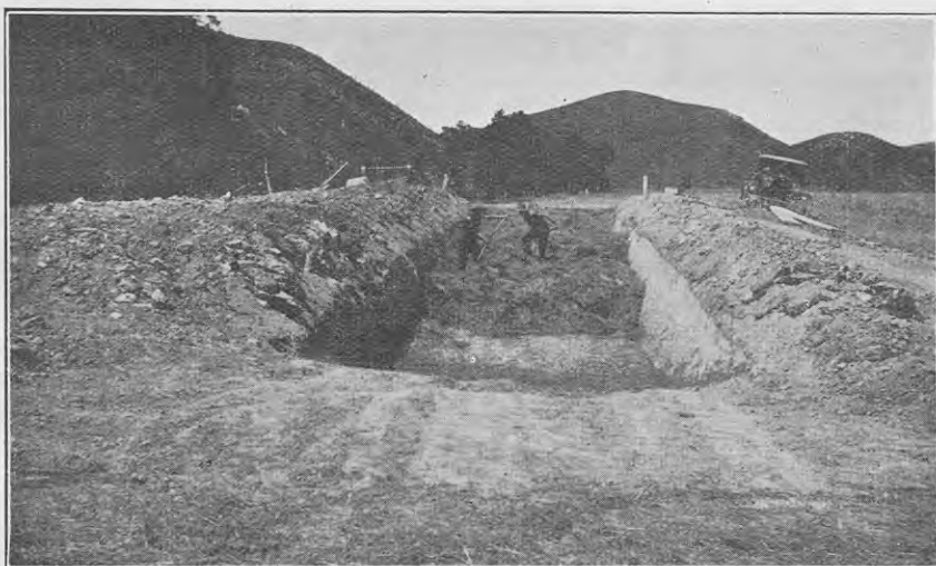
TRENCH SILO IN PROCESS OF FILLING.
