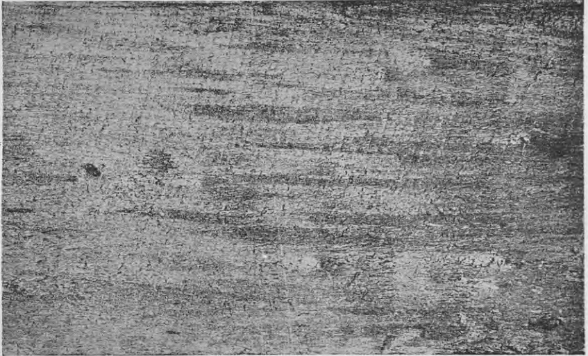
FIG. 6. TYPICAL STREAKED STAINING OCCURRING IN CLOSE-PILED TREATED STACK.
