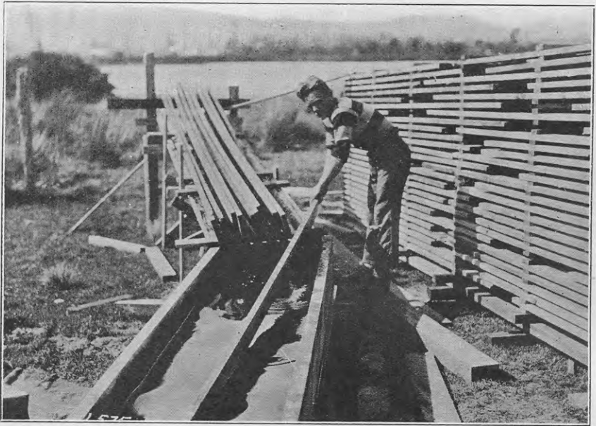
FIG. 1. METHOD OF DIPPING AND DRAINING TIMBER TO PREVENT SAP-STAIN.
