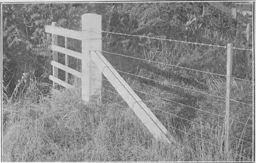
FIG. 14. 8 IN. BY 8 IN. STRAINING-POST, SHOWING METHOD OF USING DOUBLE STAYS OF 4 IN. BY 2 IN. REINFORCED CONCRETE, WITH FENCE-WIRES PASSING BETWEEN.
