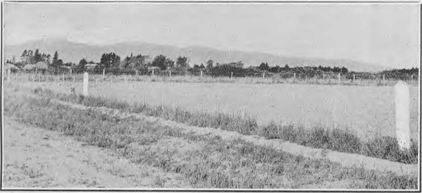
FIG. 15. SWING FENCE, WITH POSTS 6 IN. BY 6 IN. IN CROSS-SECTION, 1 CHAIN APART, AND 2 IN. BY 1 IN. WOODEN DROPPERS EVERY 6 FT.
