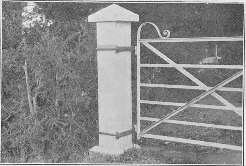
FIG. 13. 12 IN. BY 12 IN. GATE-POST MADE IN A MOULD VERY SIMILAR TO THAT OF FIG. 12.
