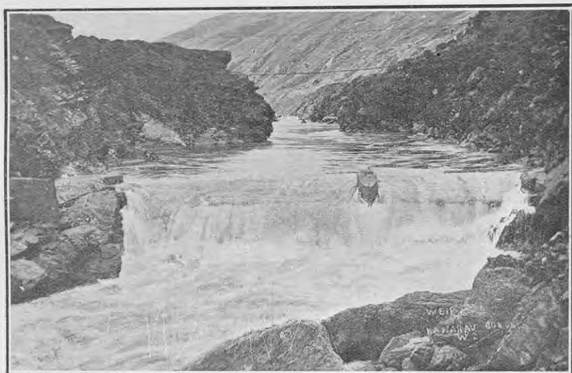
FIG. 10. KAWARAU RIVER, SHOWING CROMWELL DEVELOPMENT COMPANY'S WEIR.
