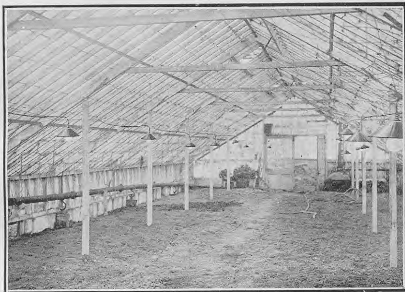
MR. LUNT'S GLASSHOUSE AT SPREYDON FITTED WITH ELECTRIC LIGHTS FOR STIMULATING GROWTH.
