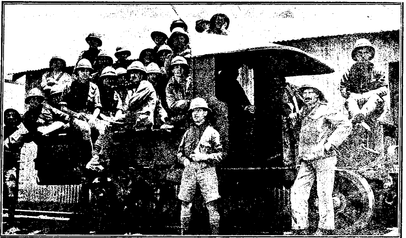
Advantages of motor transport availed of in Mesopotamia by the British military authorities. A Napier business vehicle adapted to rail traction conveying a unit of 27 men from a certain point to the front. That a moderate-powered motor lorry can transport such a body of men with ease and speed to any desired point on the railway system is, indeed, remarkable.
