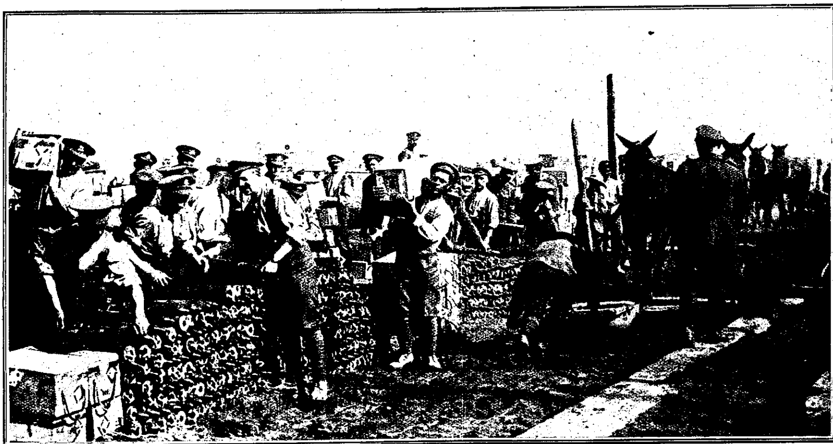
AN AMMUNITION DUMP ON THE BRITISH WESTERN FRONT. SOLDIERS ACTIVELY ENGAGED IN LEVELLING THE GROUND AND STACKING THE AMMUNITION IN READINESS FOR IMMEDIATE USE. Before stacking ammunition the ground, which has been terribly cut up by shell-fire, has to be levelled. Note the mules at work with scrapers. In the hurry up of the British advance, ammunition often arrives before the ground is levelled.
