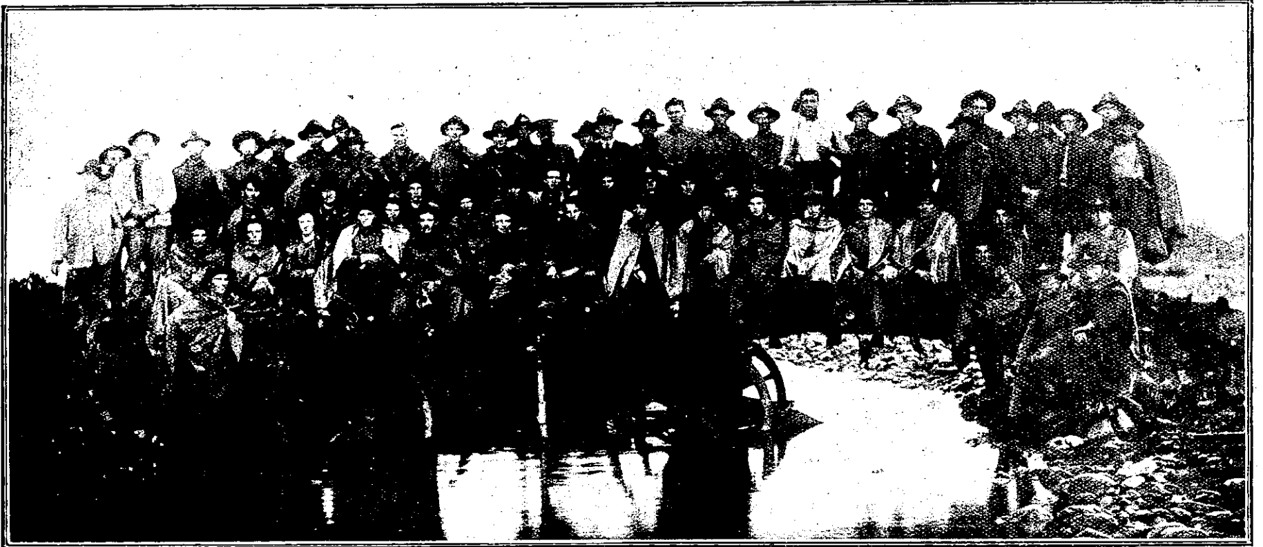
MEMBERS OF THE NEW ZEALAND FIELD ARTILLERY (30TH REINFORCEMENTS) ON AN EMERGENCY BRIDGE WHICH THEY EXPEDITIOUSLY CONSTRUCTED IN THE COURSE OF THEIR TRAINING DUTIES WHILST AT FEATHERSTON CAMP. Note the two ammunition waggons that have been used as the main supports, the wheels of same carrying all the weight. The bridge is about 25ft. long, and is supporting about 70 men.
