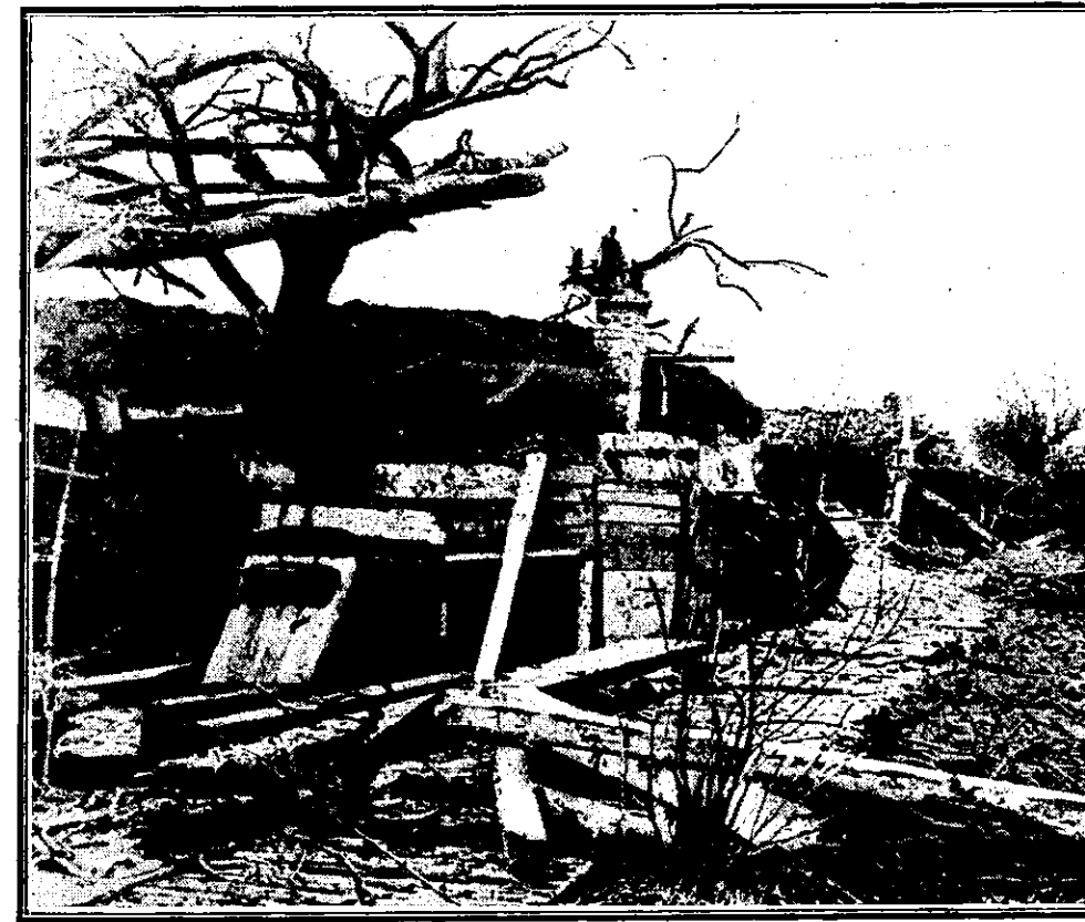
ONE OF THE MANY BATTERY POSITIONS ABANDONED BY THE GERMAN BRITISH PRESSURE. The Royal Artillery made the position untenable, the to escape from the demolishing effect of the intense s
